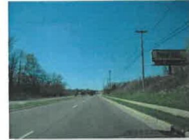
Rock Hill-Pineville Road Facing West Along Site
