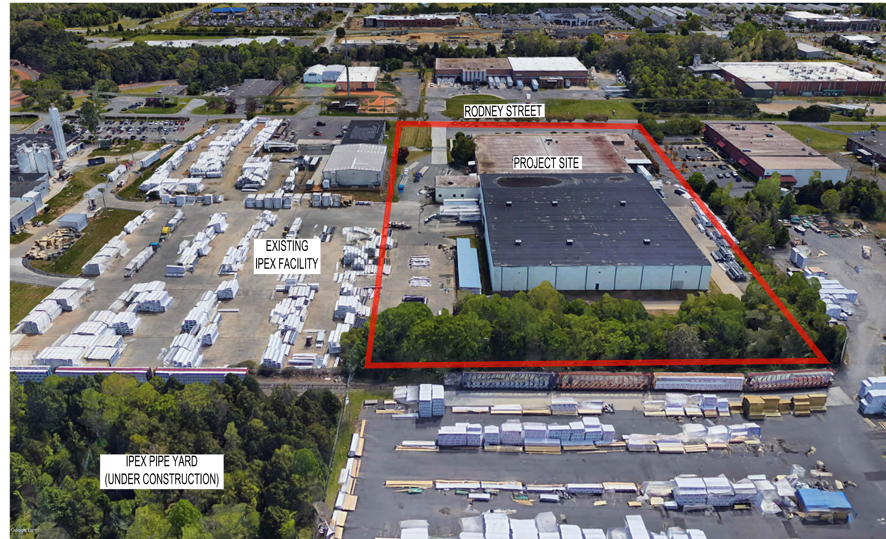
BIRDSEYE LOOKING EAST
