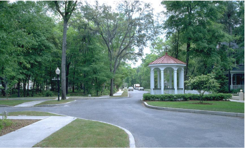
A traffic calming device that permits through-traffic but visually diverts motorists to the left
