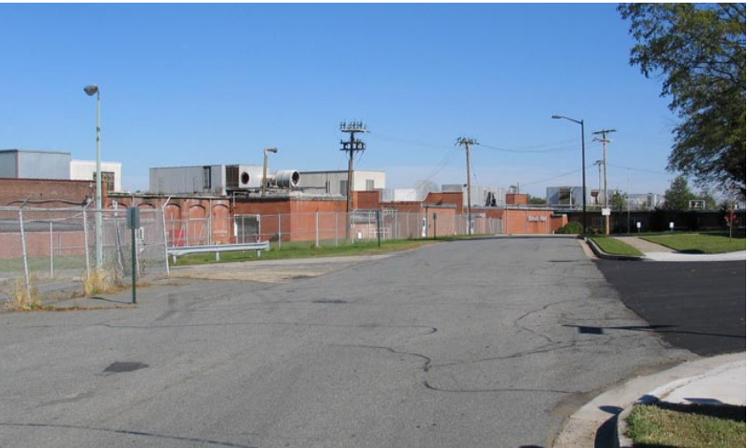
Existing conditions at the Cone Mill site
