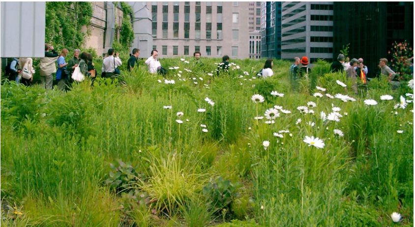
Planted garden roofs minimize stormwater runoff and reduce heat gain like this one on the Chicago City Hall
